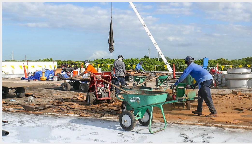
*Construction workers at the WDSrx Boca Raton, FL location apply a reflective coating during roof replacement to reduce air conditioning requirements inside the building.*
